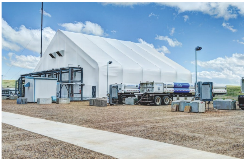
Photo caption: The picture shows the Linde engineered helium purification facility in Mankota, Canada, together with helium tube-trailers (right) for customer deliveries. (Source: The Linde Group).
